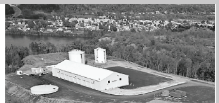
Award-Winning $65 Million River Intake & Interim Water Treatment Facility Center Township Water Authority
