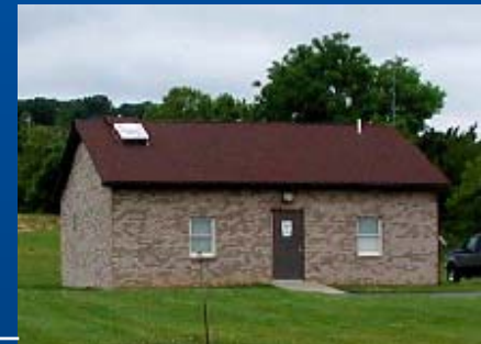
BOOSTER STATION $2M
