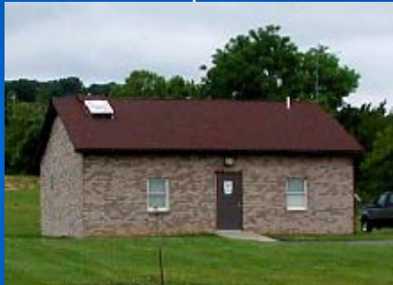
PUMP STATION $2M
